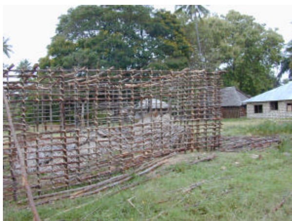
Figure 1 Building with mangrove poles
